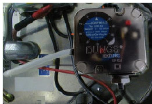
When the Giersch gas burners are put into operation, the following values have to be set at the air pressure controller LGW 10A2
